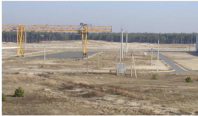
SRW-1 disposal facility
