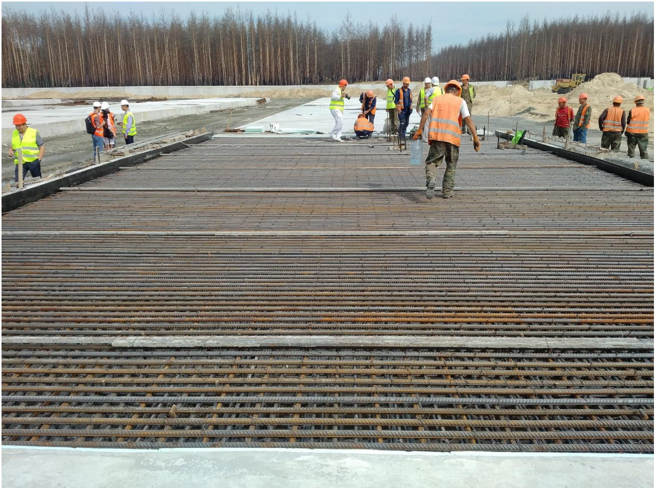
Activities at CSFSF construction site
