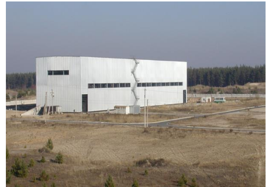
SRW-2 disposal facility
