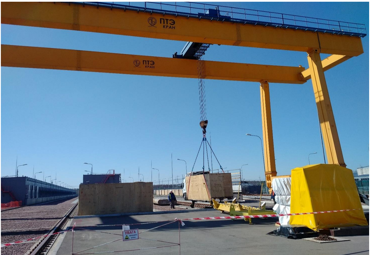
Acceptance of a double-walled dry shielded canister at ISF-2 site. Storage area is on the left in the background
