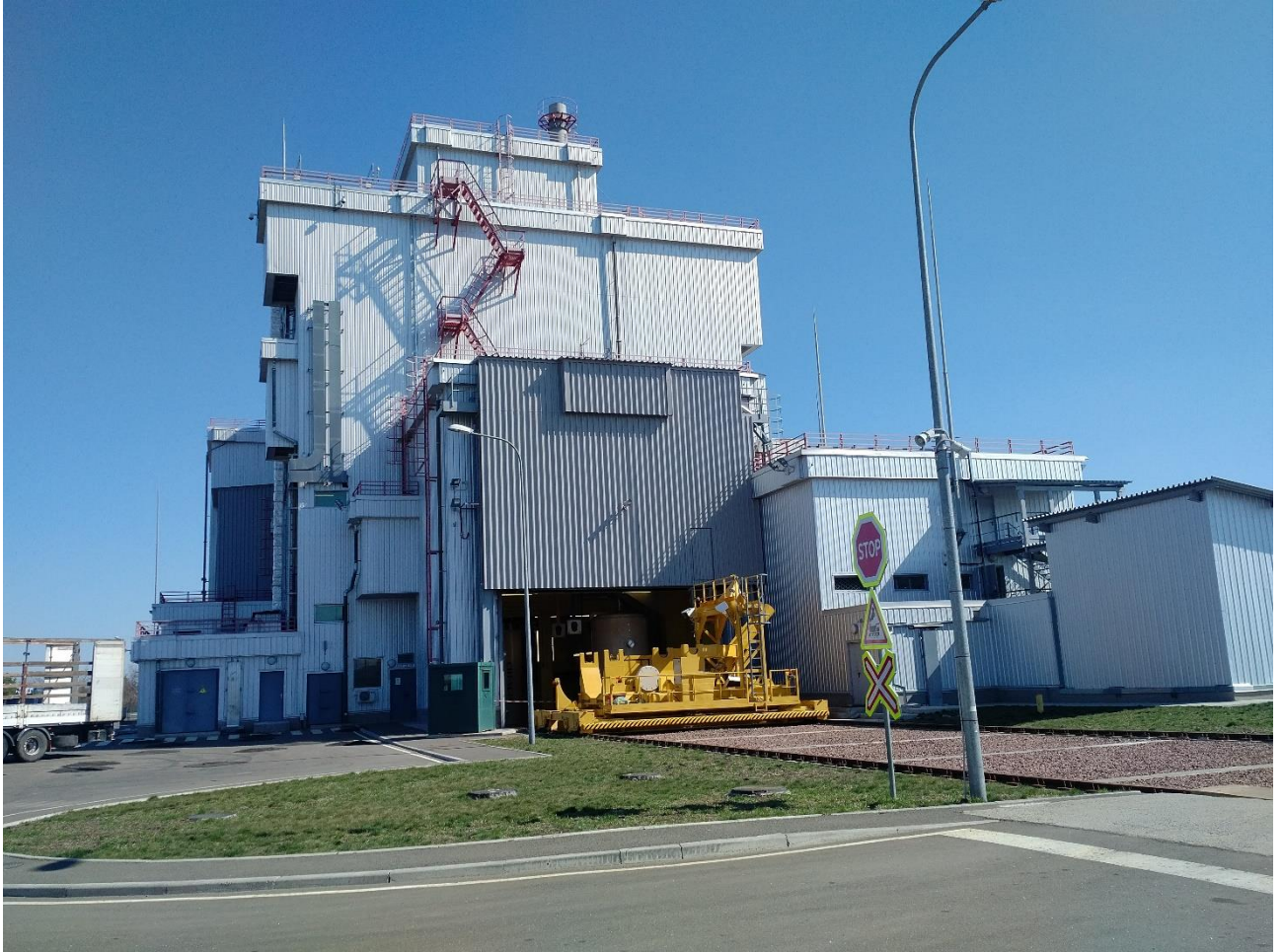
Spent fuel processing facility (ISF-2 SFPF)
