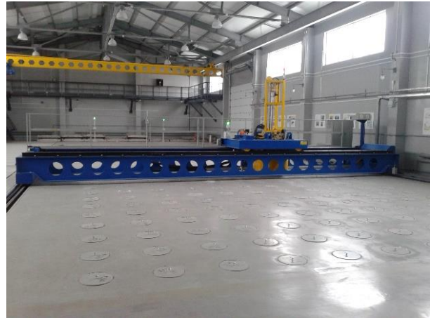
Storage area for disused radiation sources in CLTSF
