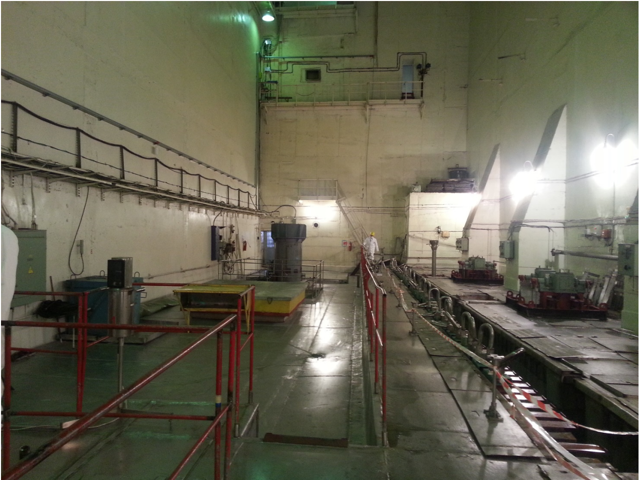
ISF-1 room with the cooling pool canyon with damaged SNF
