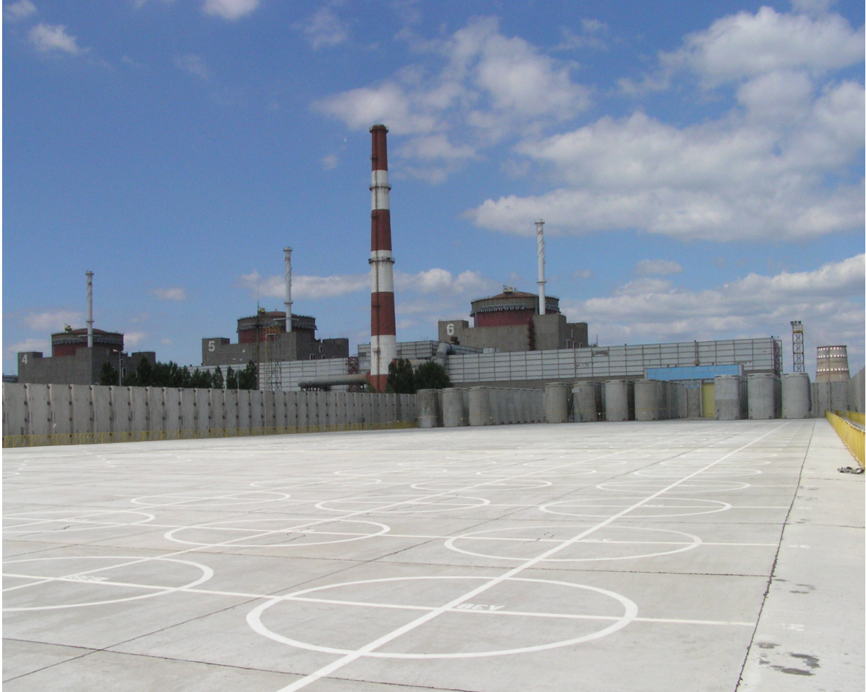
Zaporizhzhya NPP Stage 1 with a capacity of 100 VSCs was commissioned in 2001 and Stage 2 with a capacity of 280 VSCs was commissioned at the end of 2011.
