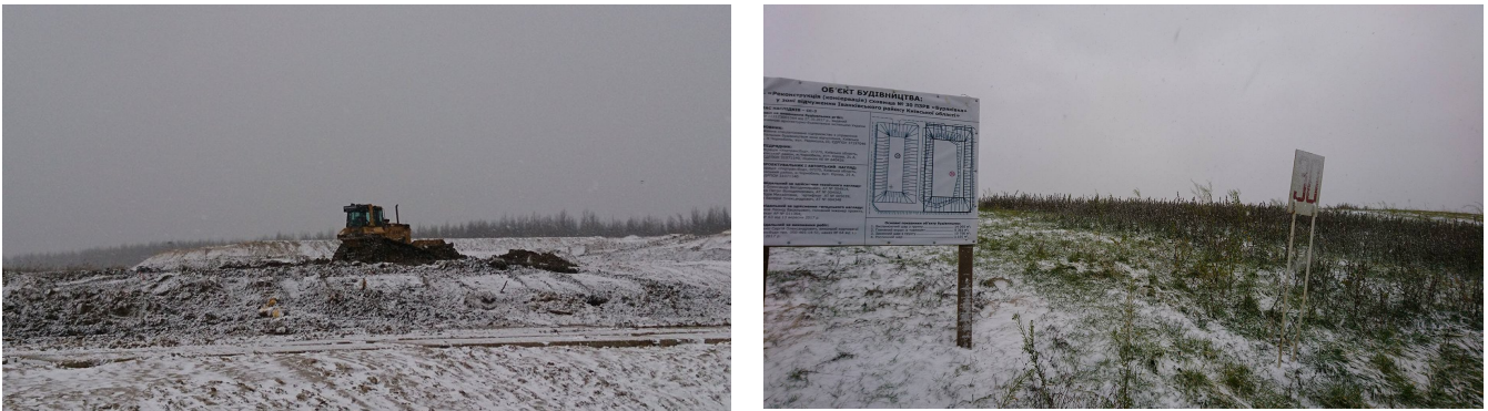
Closure of Buryakivka RWDS trenches
