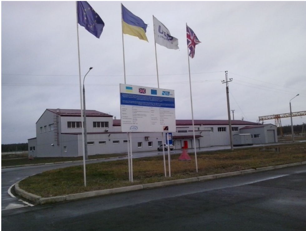
Centralized long-term storage facility for disused radiation sources (CLTSF)
