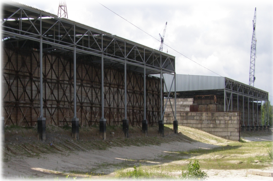
Pidlisny RWDS modules A-1 and B- 1 after safety improvement project
