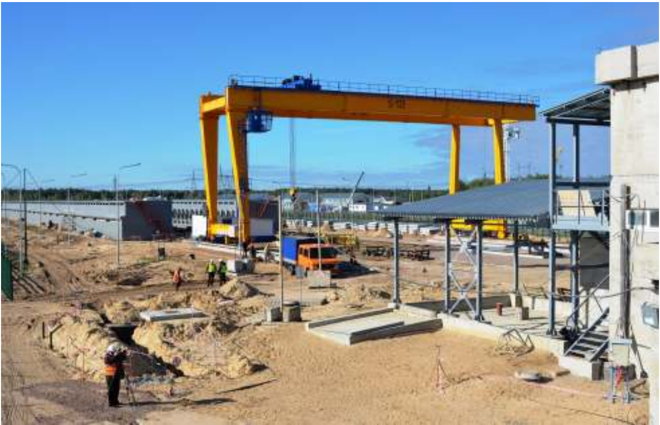
ISF-2 construction site
