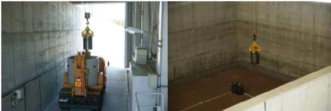
Figure 7.3.2. Loading of the first radwaste package lot in ENSDF
