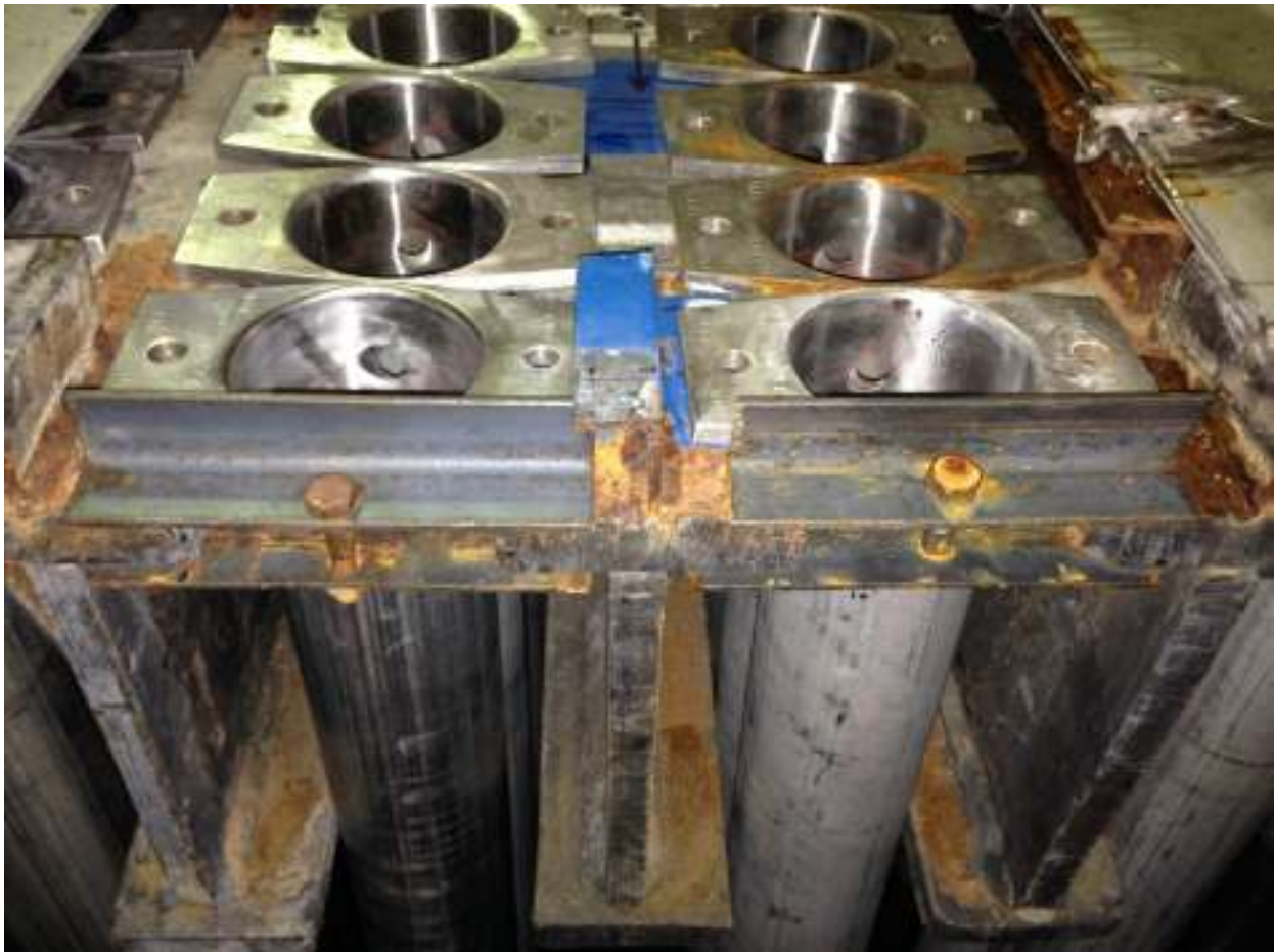
Figure. 5.3.4. Storage of canisters with spent nuclear fuel in ISF-1
