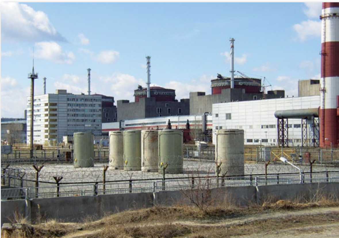
Zaporizhzhya DSFSF site. First containers
