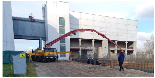
Photo 7. Pouring the foundation for KhNPP RWTP
