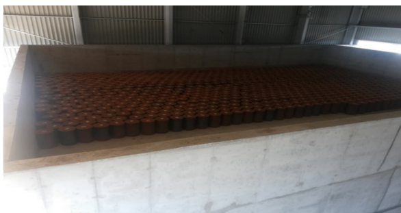
Photo 11. Completion of the fifth layer in ENSDF module D1
