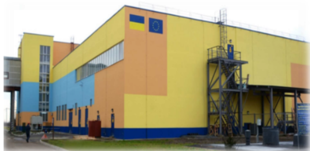
Photo 6. RNPP RWTP building
