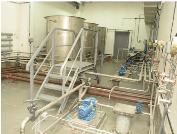
Photo 4. Installation for centrifugation and purification of radioactive oil at RNPP
