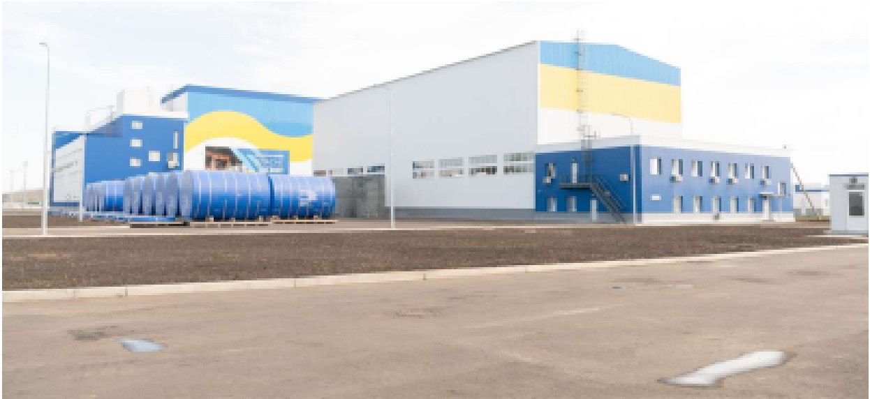
Photo 2. CSFSF site (maintenance building, acceptance building)
