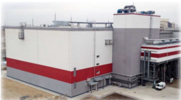
Photo 5. ZNPP RWTP building
